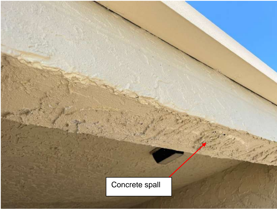
East Side Concrete Beam at 4 th Level Stairwell
