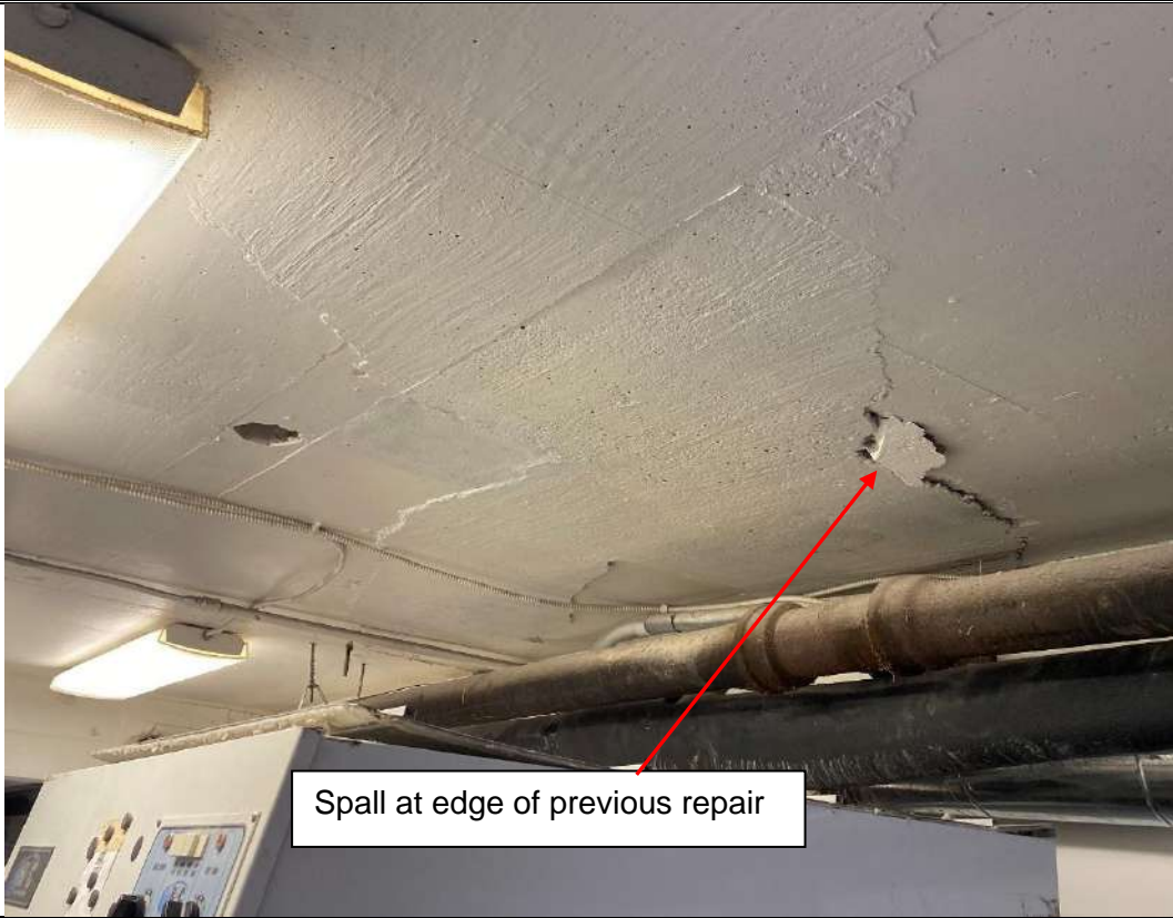
Mechanical Room Overhead
